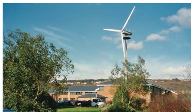
Community building with small turbine
