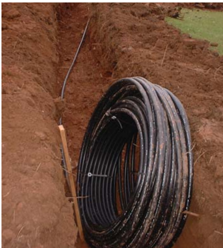
Installation of a ground collector
